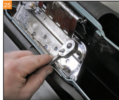
Final tighten the first #8 bolt installed.
